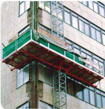
Platform can be turned 90° to the side of the main platform
